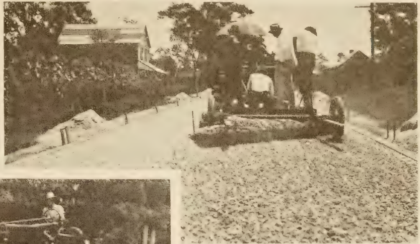
BELOW: THE DRAG PROVED VERY SATISFACTORY FOR SMOOTHING THE SURFACE AFTER THE MIXING OPERATION WAS COMPLETED
